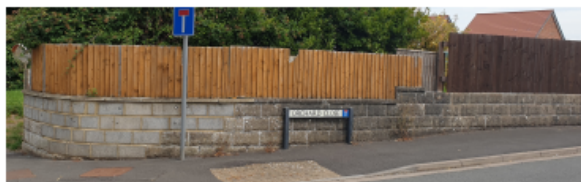
EXISTING WALL VIEW FRONT (NORTH-WEST) (B)
